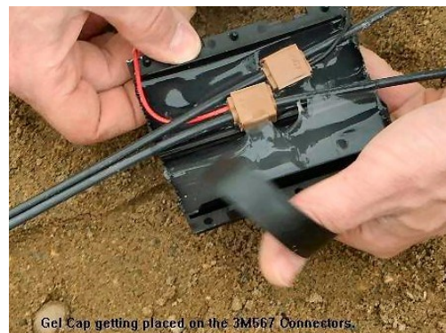
Gel Cap getting placed on the 3M567 Connectors.
