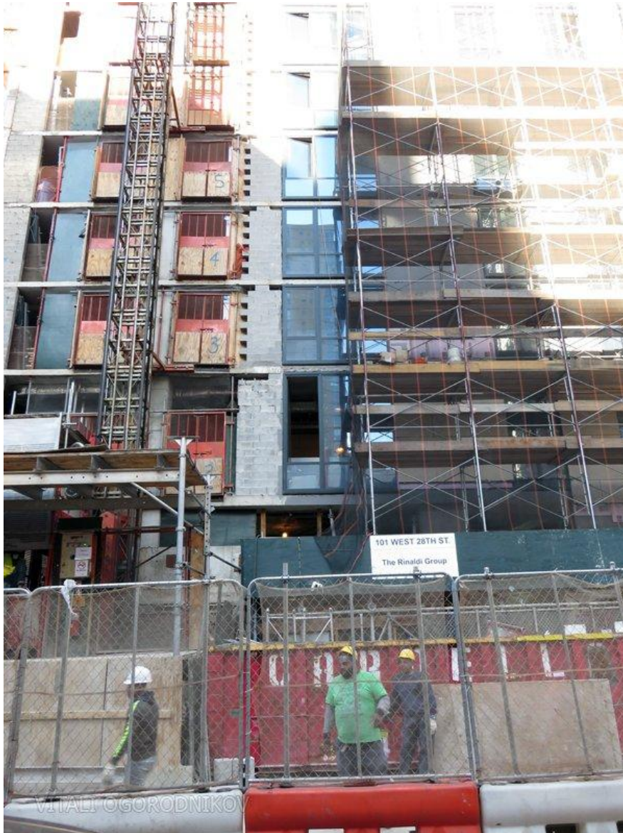
Hyatt House base under construction
