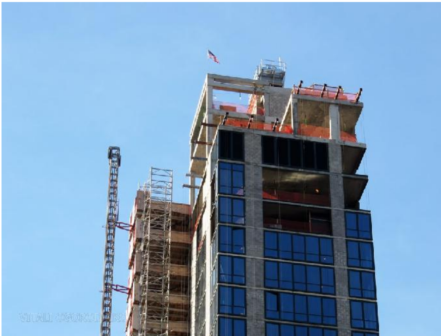
Building crown, east façade
