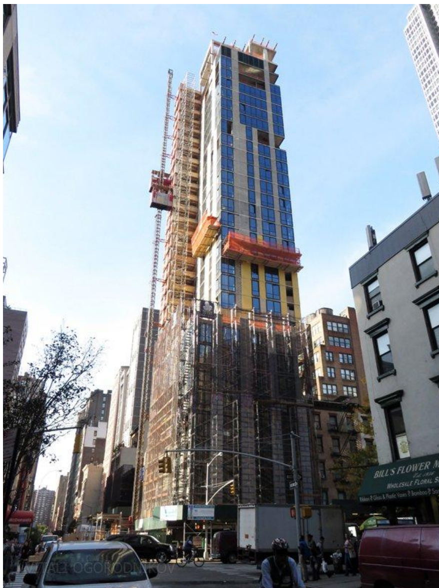
Hyatt House nears exterior completion
