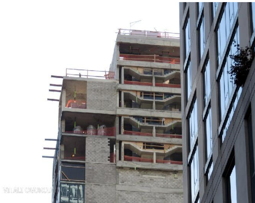
Building crown, north façade
