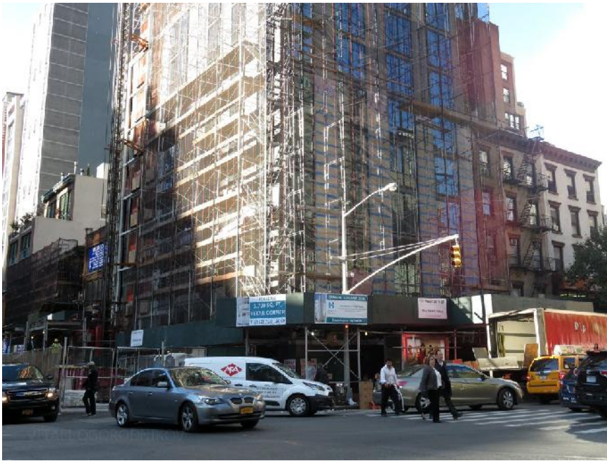
Hyatt House base under construction
