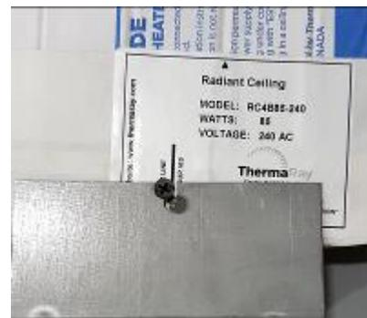
10. Fasten the enclosure securely using the gypsum screw provided, screwing through the enclosure, through the heating panel and out through the screw hole on the upper side of the MC-2 body.
